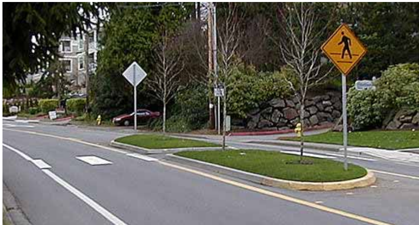
Example of a pedestrian refuge median
